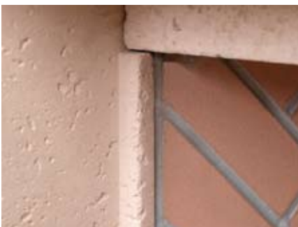
The transition from refractory to the exterior surround is seamless
